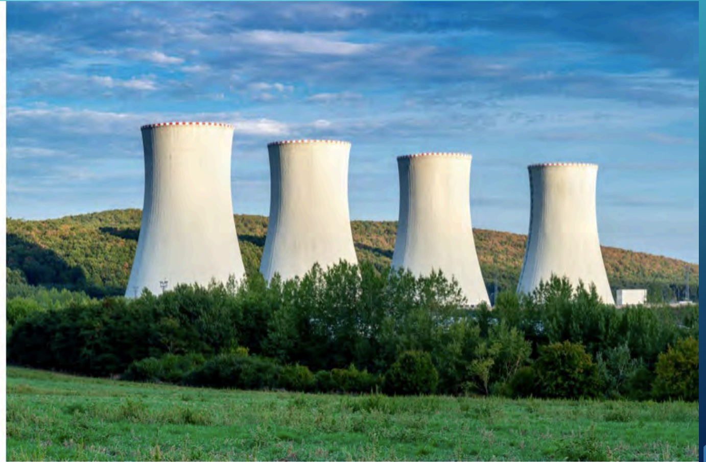
The Mochovce nuclear power plant in Slovakia. PHOTOGRAPH: STEFAN SUTKA/GETTY IMAGES
